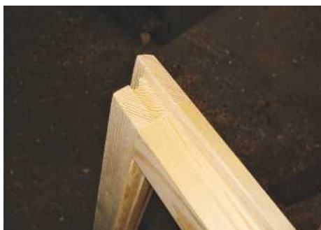
▲ Pic.24 ...to create the channel that prevents the ingress of water
